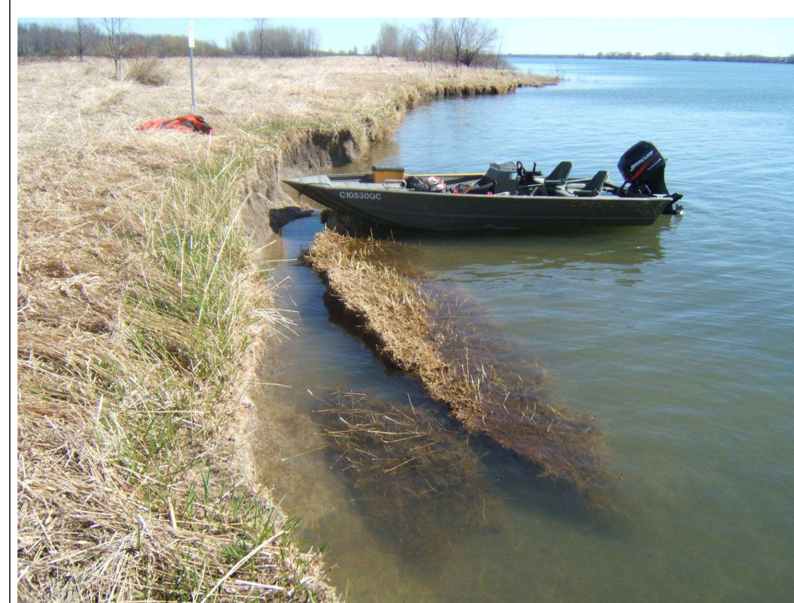
Verchères Station showing caved-in banks in spring
